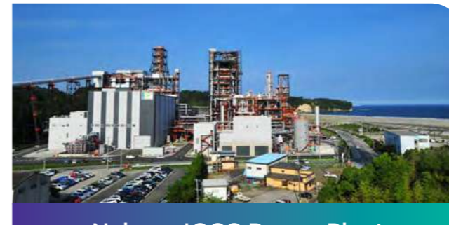
Nakoso IGCC Power Plant
