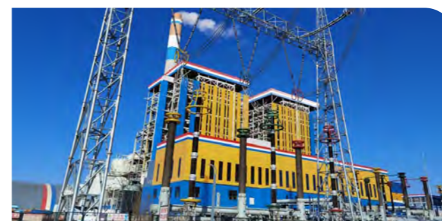
Shanxi Lu Guang Power Plant
