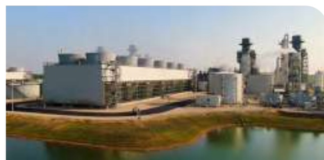
Temple I CCGT Power Plant
