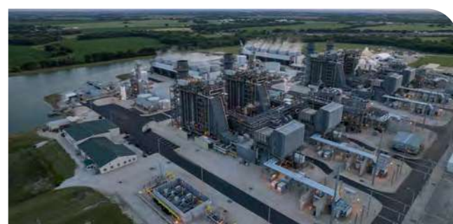
Temple II CCGT Power Plant
