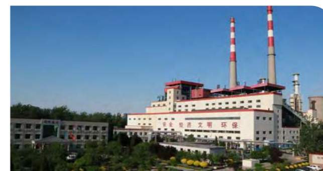
Zhengding Combined Heat and Power Plant
