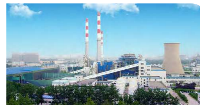
Zouping Combined Heat and Power Plant
