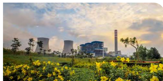
HPC Power Plant
