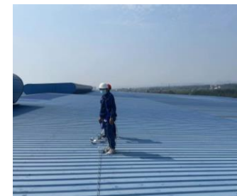
Solar rooftop at coal yard roof
