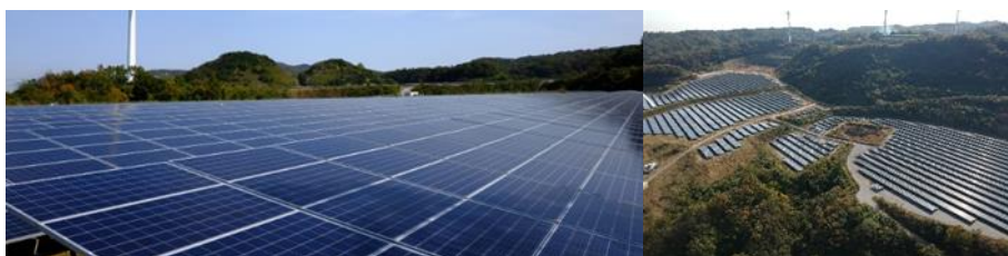
Solar panels at Awaji Solar Power Plant, Japan
